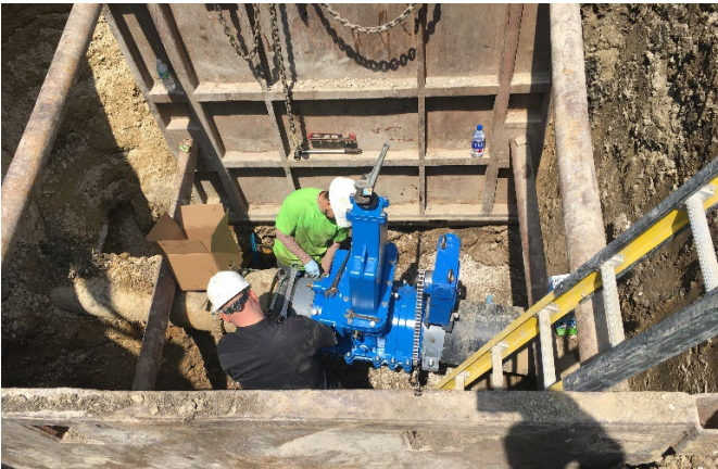
2017 Insertion Value Installed on Existing 14” Force Main
