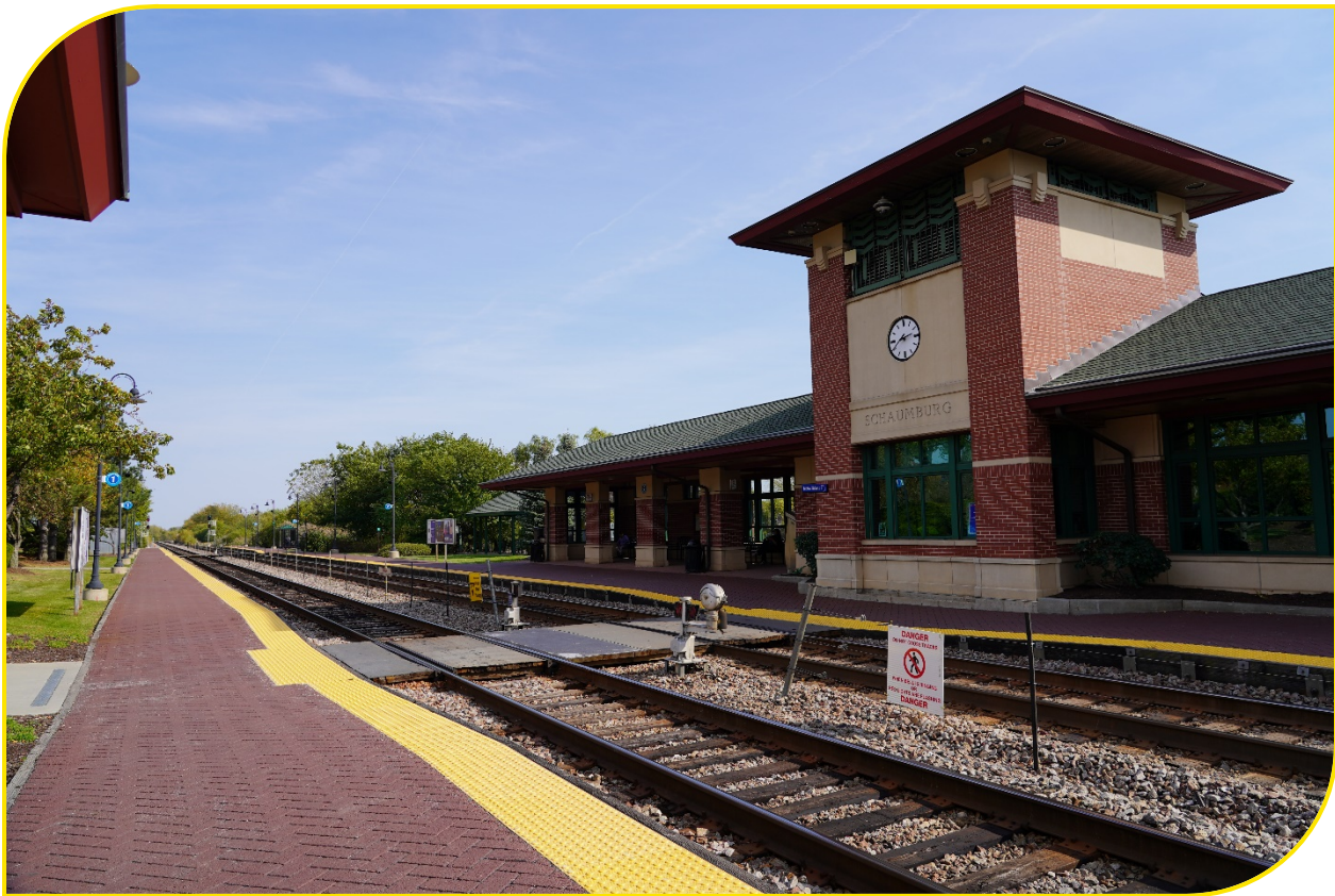
Schaumburg Metra Station serviced by the village's Commuter Lot
