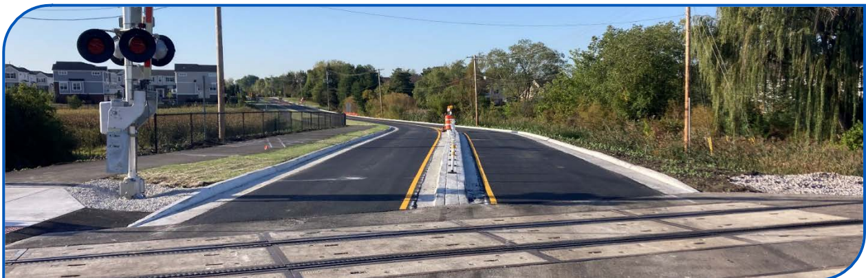
Work on Rodenburg Road Reconstruction Project Completed in FY 24/25
